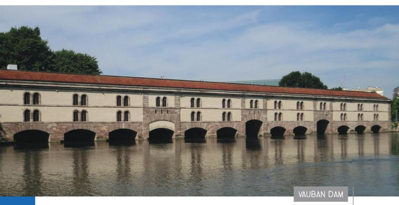
Desalination of the downstream facade of the dam, located in Strasbourg, using a desalination compress from the Advectum® range.
